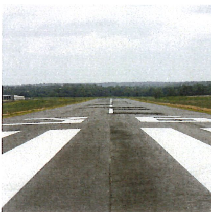
Bristow Relocate Runway 18/36
