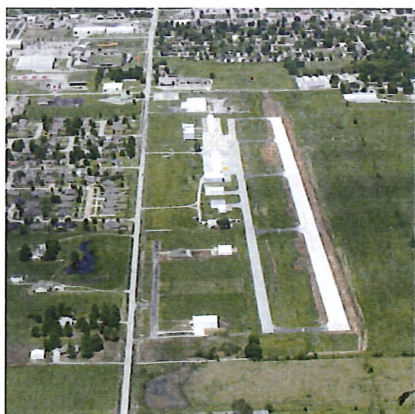
Skiatook Reconstruct Runway 17/35
