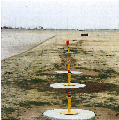
Altus Rehabilitate Runway Lights
