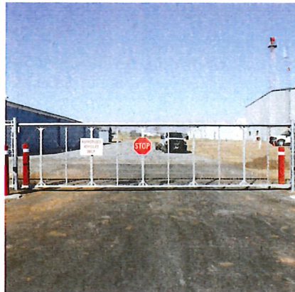
Duncan Install Perimeter Fencing and Gates
