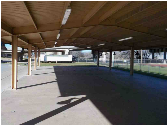
Subject Covered Parking - North Side
