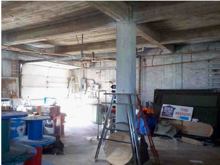
Subject Warehouse/Strg Area - First Floor
