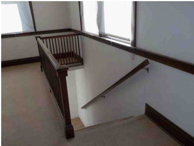
Subject Stairwell Leading from Second Floor to First Floor
