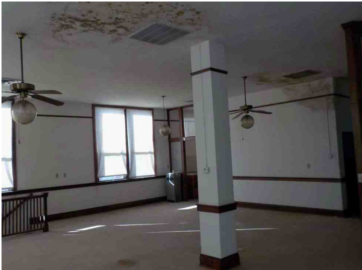
Open Office/Lobby Area - Second Floor (2 of 2)
