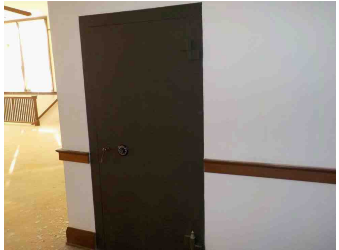
Subject Vault - Second Floor
