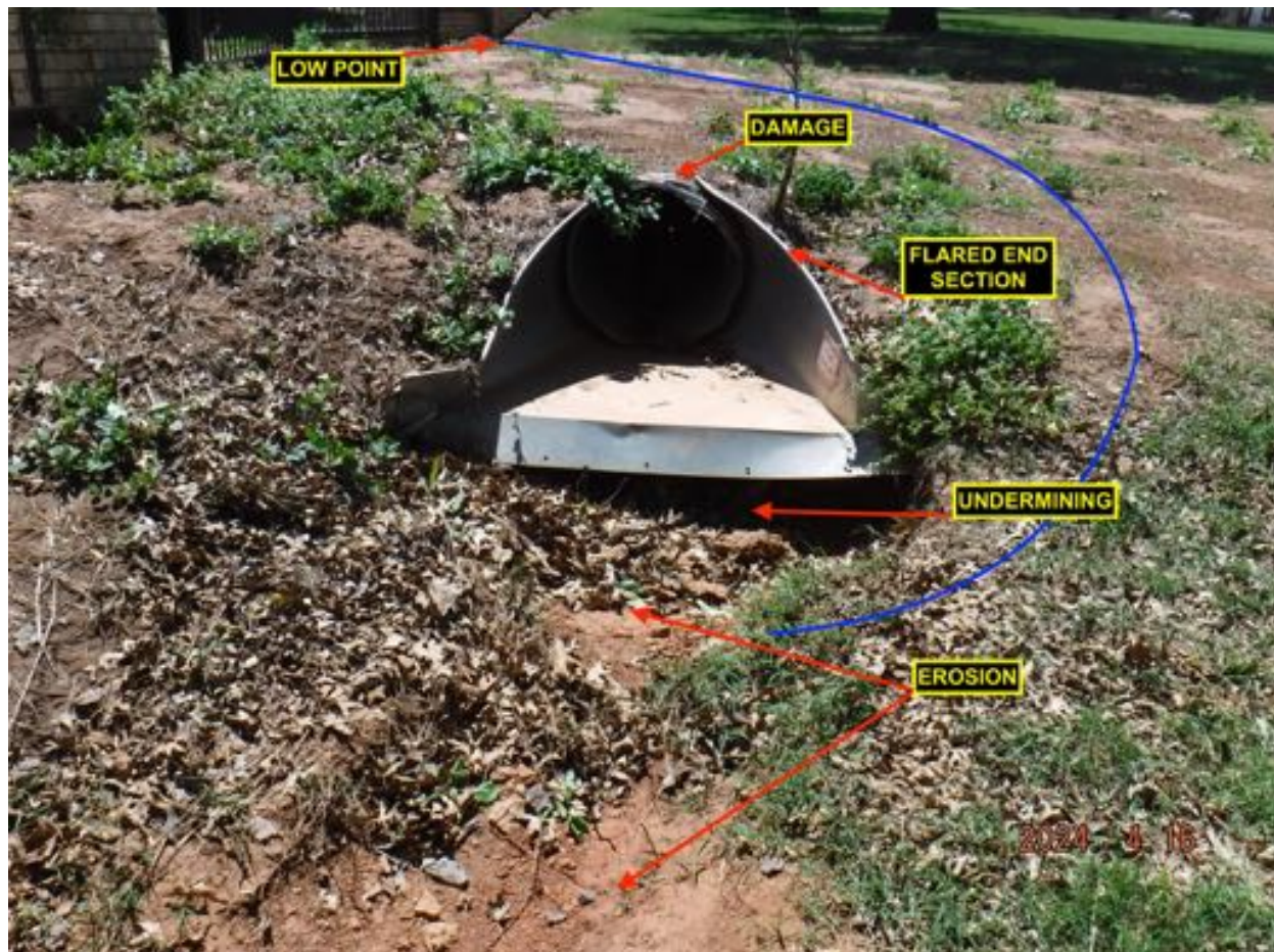
Figure 2: OUTLET CONDITIONS OF THE 24" CMP
