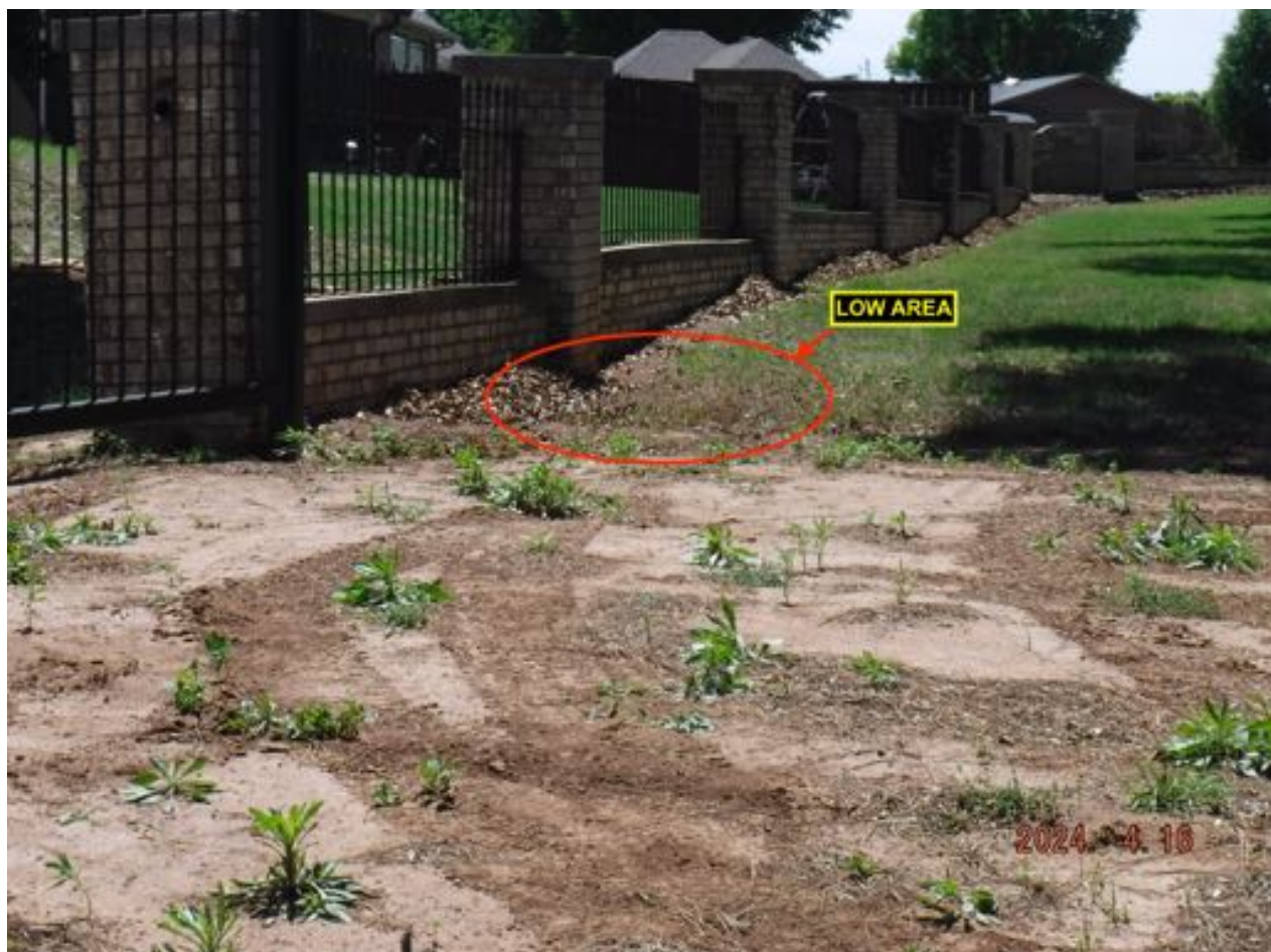
Figure 3: CLOSE UP OF LOW AREA SOUTH OF THE 24" CMP INSTALLED
