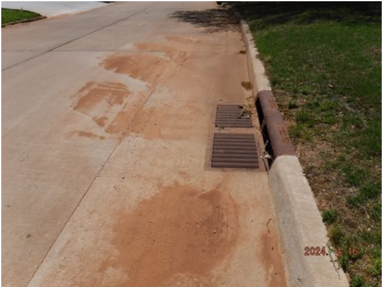
Figure 6: CATCH BASIN 507-FEET DOWNSTREAM OF THE CATCH BASIN SHOWN IN FIGURE 5.
