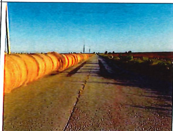
Looking south along 2-lane asphalt drive
