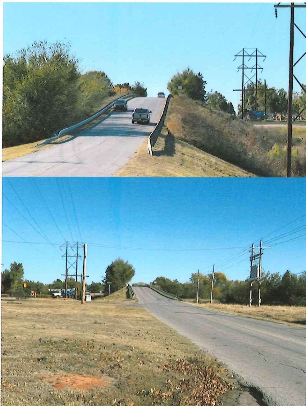
Fig. 2 — I-44 Overpass: No Shoulder, Limited Visibility
