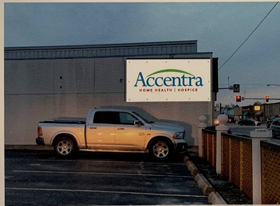
5' X 10' ALUMAPANEL , DIGITAL PRINTED U.V. VYNAL INSTALLED EAST SIDE WALL MOUNT.
